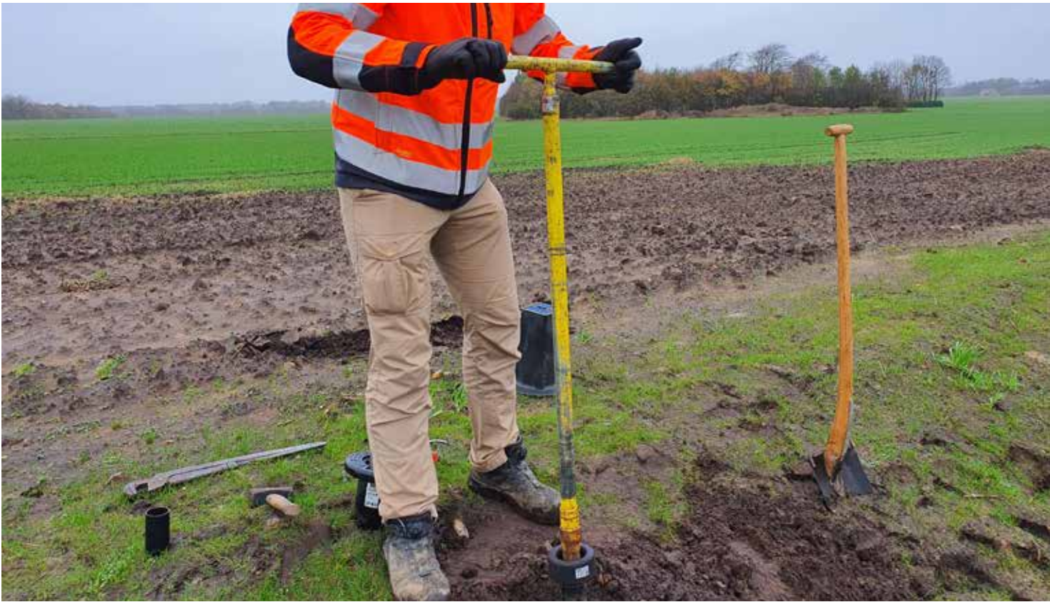
The VIDI Positioner is calibrated and ready to detect the position of the gate valve.
